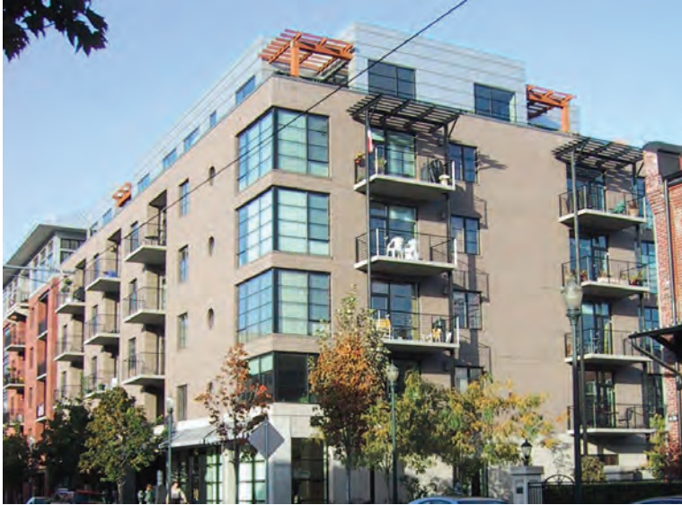
Variations in rooftop design help create interesting skylines
