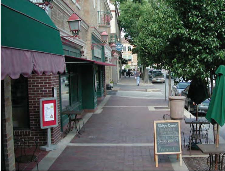
Driveway across sidewalk identified by material change
