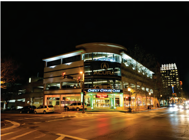
Building designed to screen service and repair areas from the street
