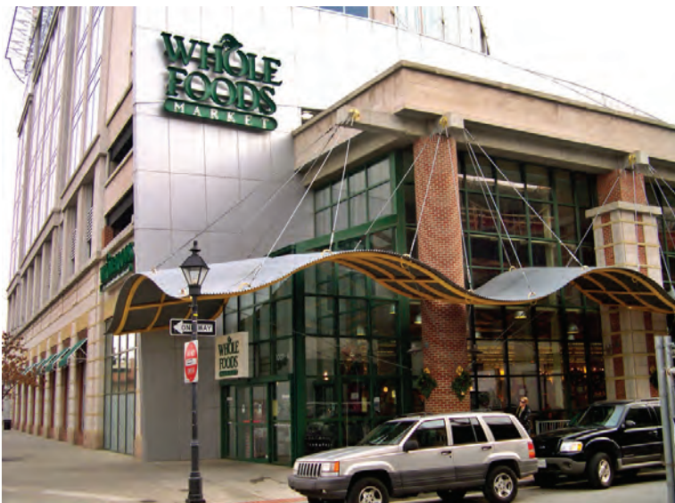
Use of structural element to anchor the corner for a commercial development
