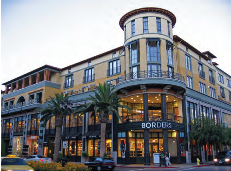
Iconic building and corner treatment
